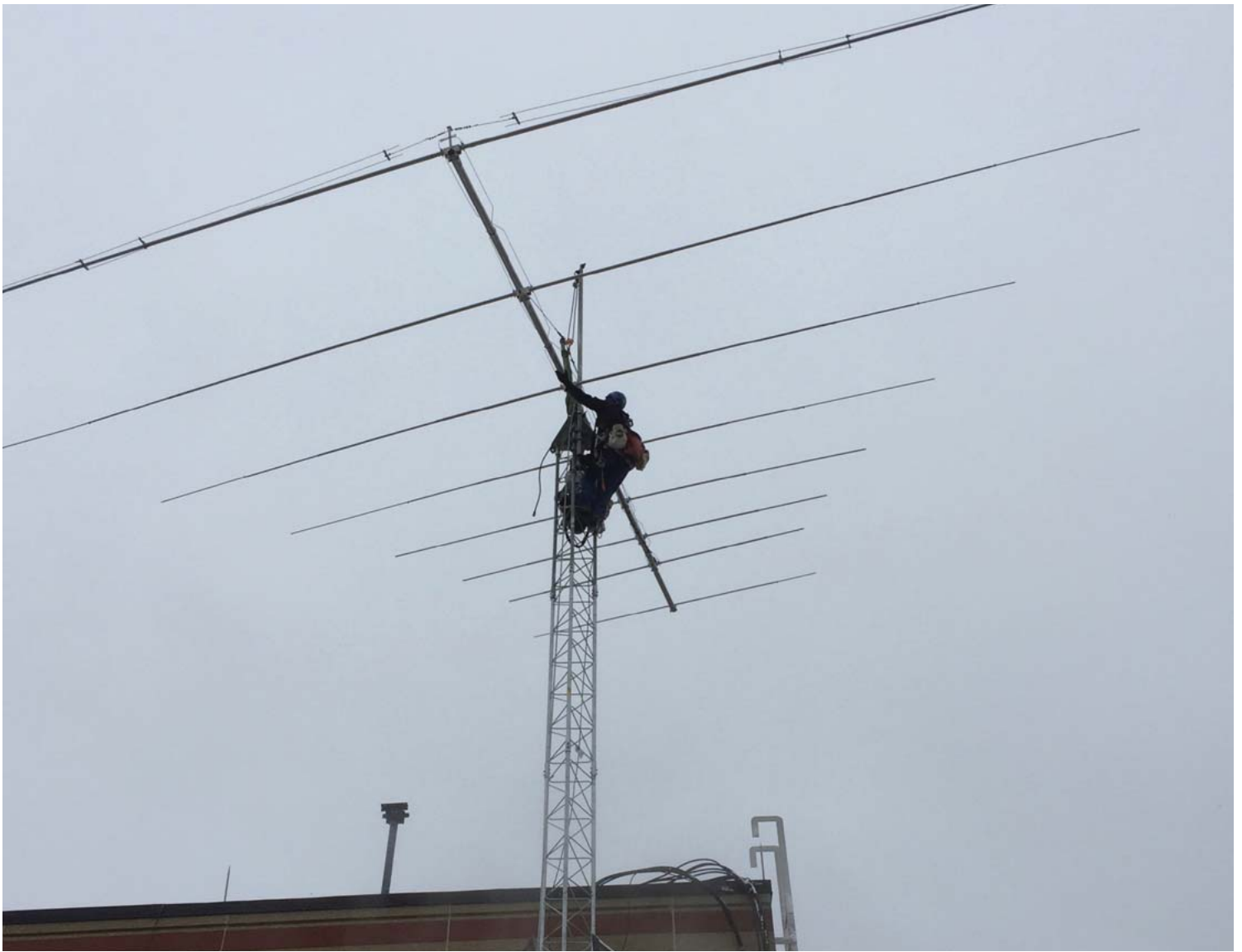
The HF log-periodic dipole array in this photo is one of the antennas serving the SHARES HF Radio Program Office near DHS Headquarters in Washington, D.C. (Photo courtesy of Department of Homeland Security)
